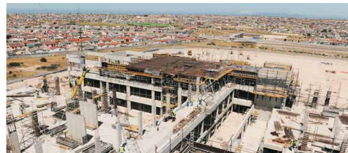
Construction of the District Hospital in Khayelitsha CBD
