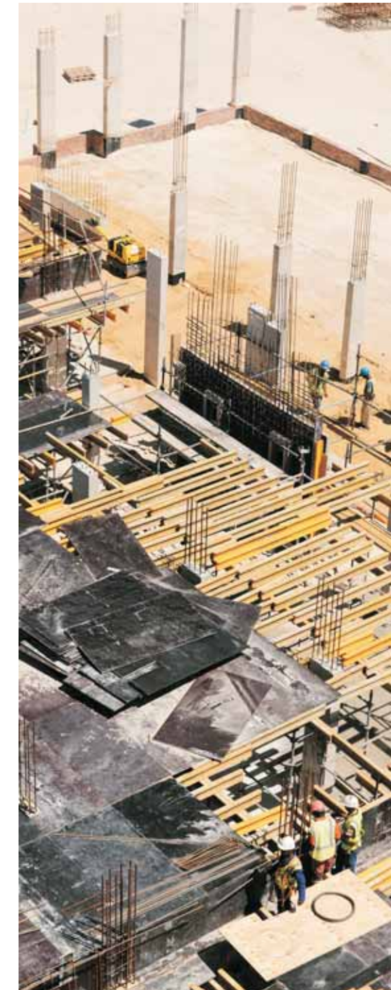
Construction of the District Hospital in Khayelitsha CBD
